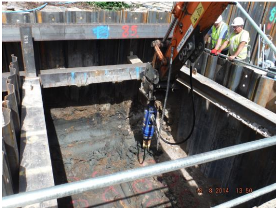
Piling probing and clearance works
