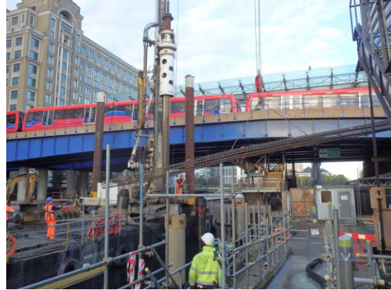
Rebar cage installation
